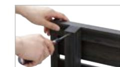
Place the cover caps on the posts and fasten with screws
