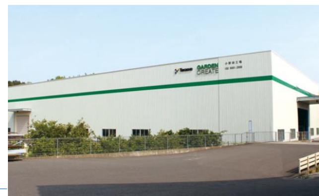
Garden Create Headquarter and Wakayama Factory ISO 9001 Certified Factory
