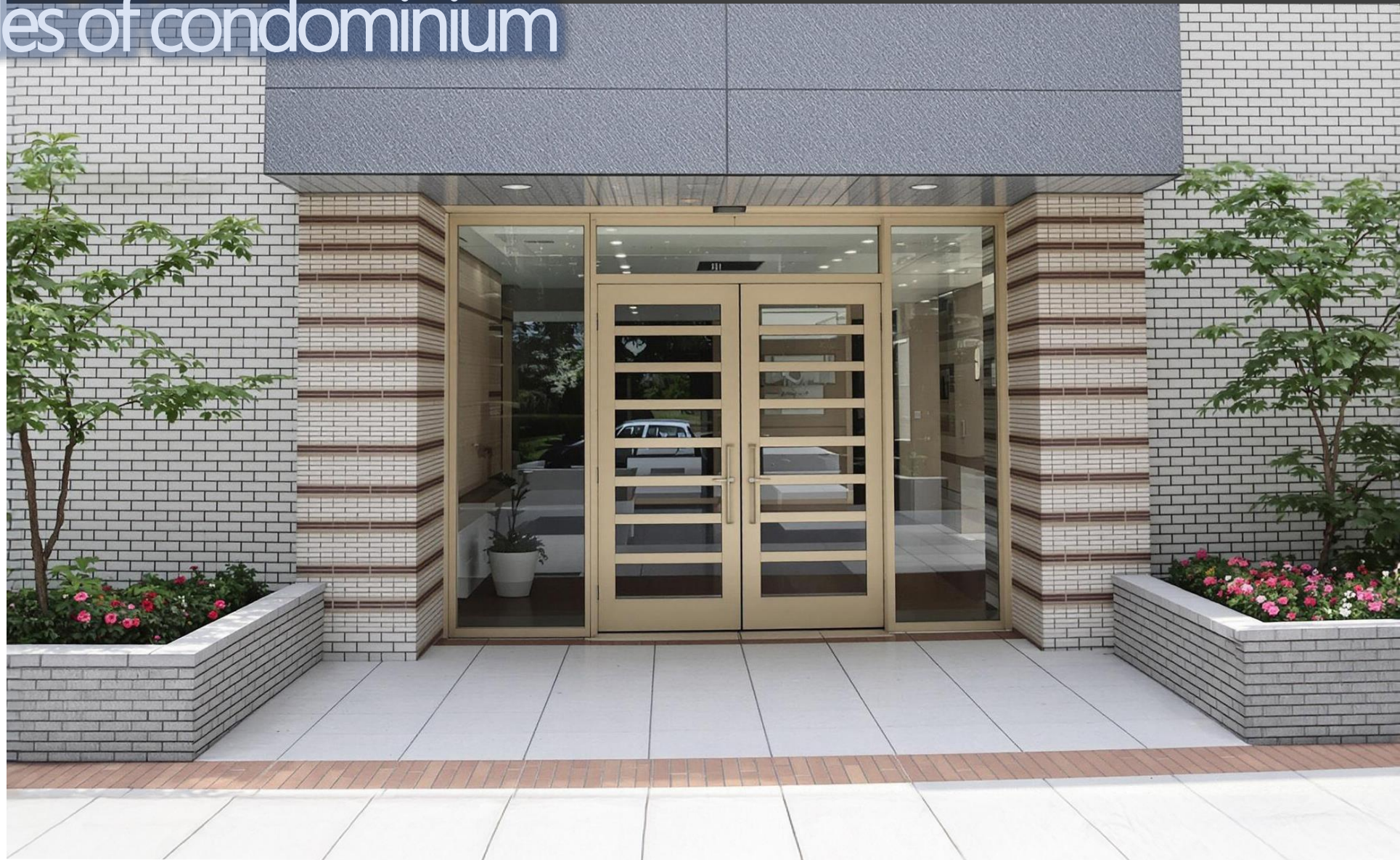
Niwa Plus case study: Condominium façade
