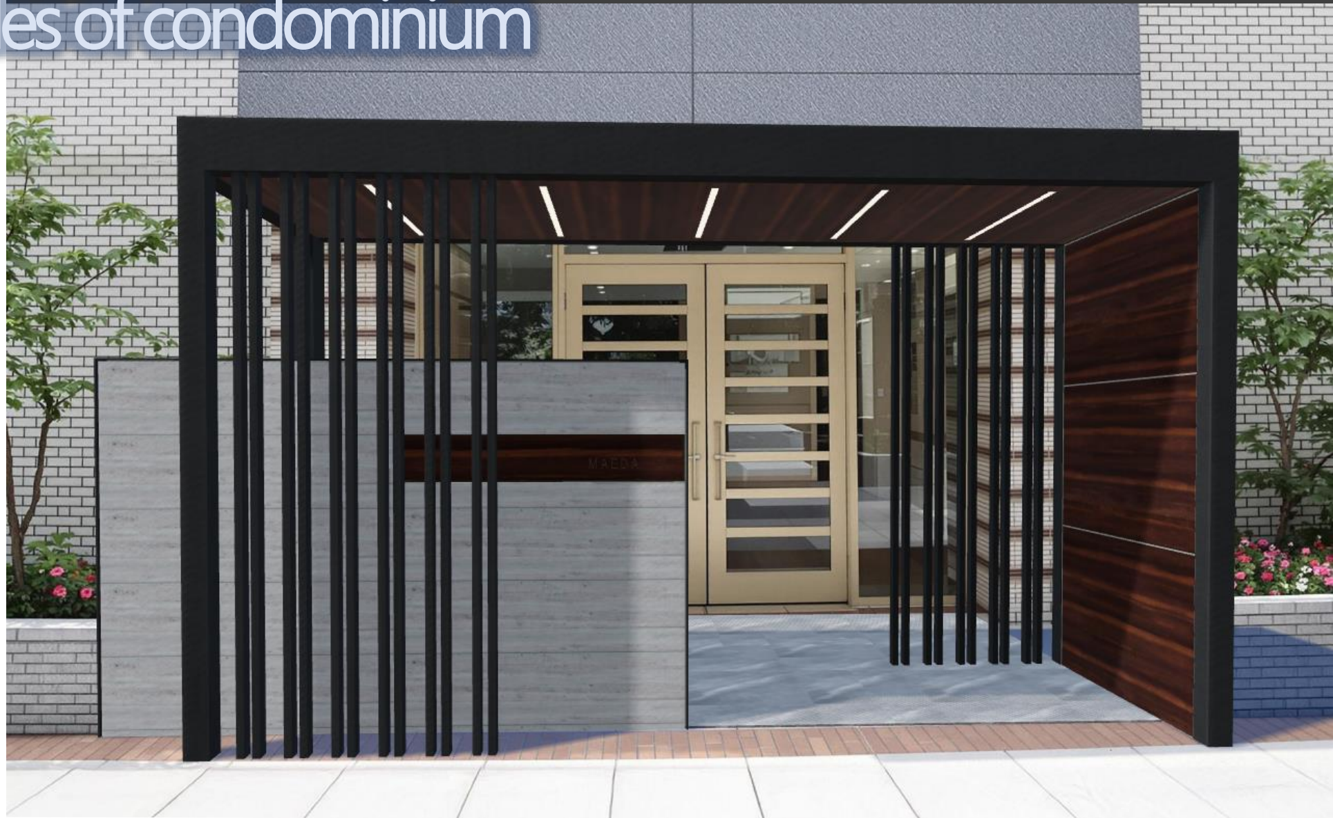
Niwa Plus case study: Condominium façade
